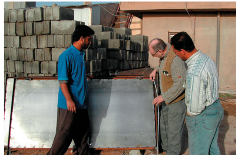
Construction of a new laboratory door.
